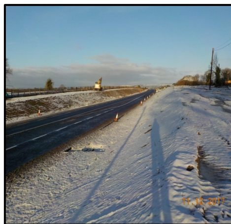
Callan Road Realignment Scheme
