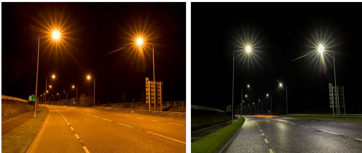
N77 Kilkenney Ring Road before and after
