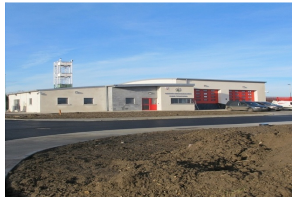
Construction of the new fire station for Graiguenamanagh taking shape
