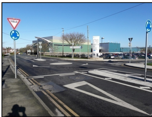
Low Cost Safety Improvement Works on the Freshford Road
