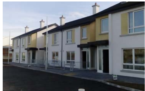
7 units at Newpark (The Haven) , completed in 2017 under a turnkey scheme
