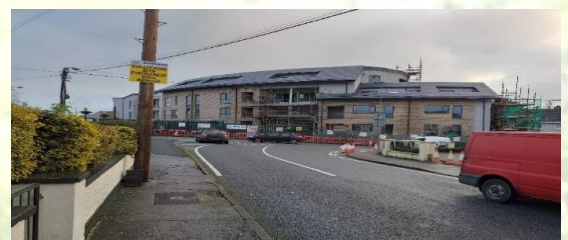
27 Units at completion stage at Walkin Street, Kilkenny
