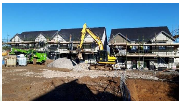
17 units under construction at Breagh Place, on Main Street, Piltown
