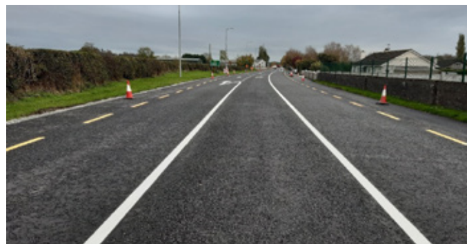
N77 Oldtown to Ballyragget – Finished Pavement
