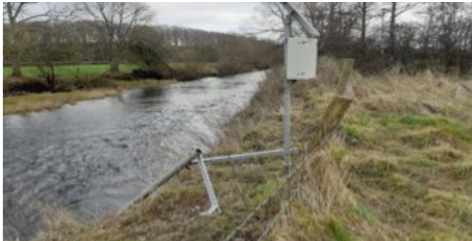
Water Quality Monitoring Station
