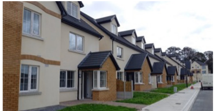
Seville Rise, Margaret's Field, Callan Road, Kilkenny City. 40 units completed January 2021 – AHB Turnkey – Respond Housing
