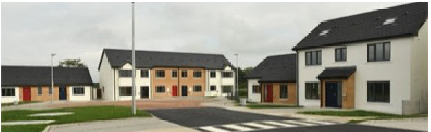
Station Avenue Phase 2, Ballyragget, Co Kilkenny. 22 units completed June 2021 – KCC Direct Build. Designed by CJ Falconer and Associates Contractor:- Thos. Kelly & Sons
