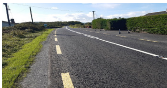
N76 Riversfield to Ahanure North – Finished Pavement
