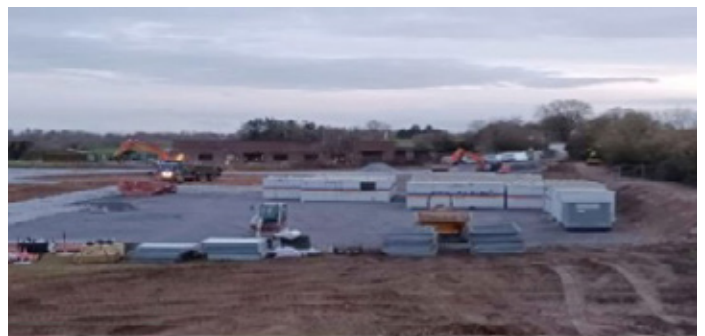
Compound setup including Safety, health and welfare facilities, offices, material storage and car parking
