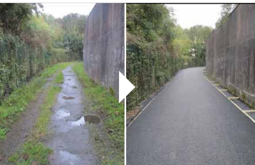
Before and after: New cycle way at O'Loughlin Road, Kilkenny
