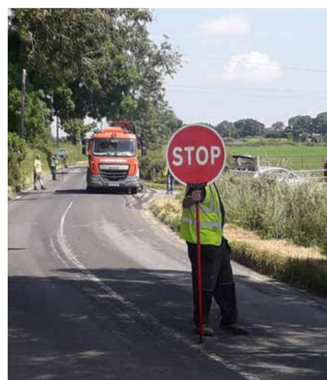
Kilkenny County Council Road Maintenance - North Callan Roads Crew
