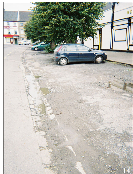
Photo 14: View along south side of The Square - road surface is in poor condition. The area would be suitable for new pavement and kerbing with delineated parking bays and additional tree planting.
