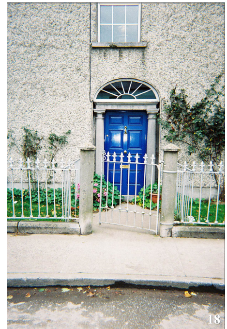
Photo 18: Ballyragget displays a significant number of fine town houses, of two storey, two storey over basement and/or three storeys high. Most are designed in the Georgian style. Note the attractive Ionic columns, fanlight window and limestone pillars in this example.
