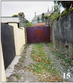
Photo 15: There are few examples of traditional paving types around the town - here stones are used to give a cobblestone effect.
