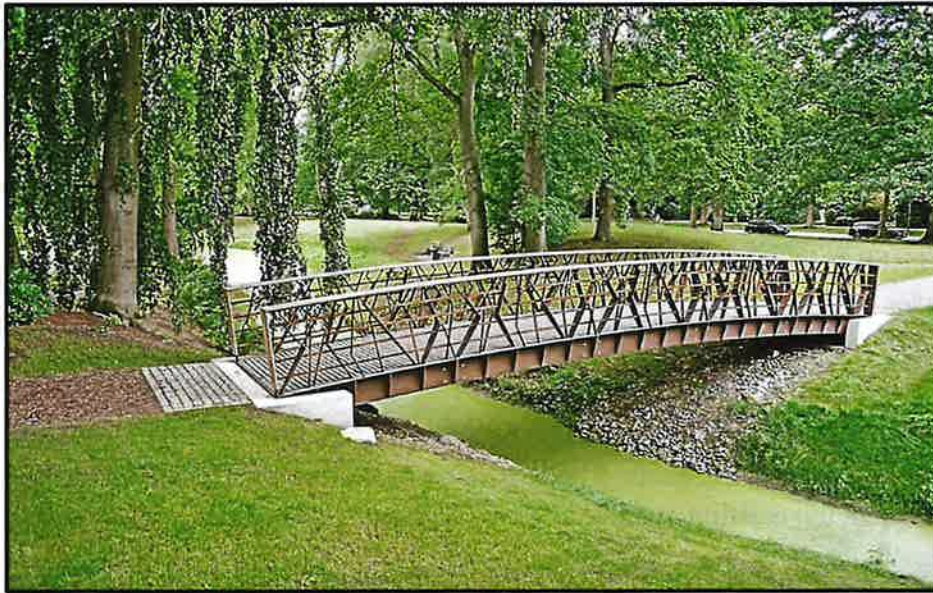
PLATE 2 - STEEL BEAM BRIDGE
